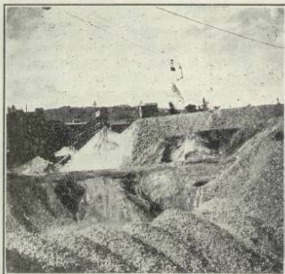
DUMPING WASTE AT THE AJAX TO MAKE TAILING DAM.
